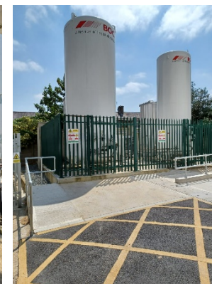
VIE Oxygen Plant - creation and installation of two new oxygen tanks and supplies to main ITU wards in C block.
