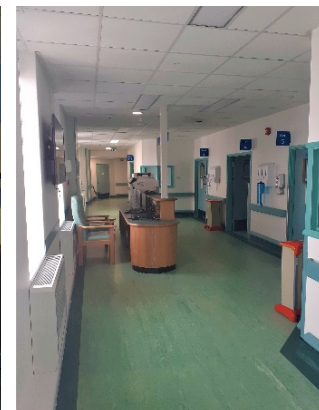
A6 and B6 ward refurbishments , converting the wards from standard medical wards to new specialist renal wards.
